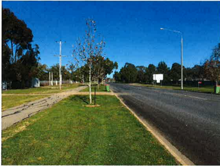
Figure 8 – View south along the Federation Avenue frontage of the subject land. Not the wide road reserve and road infrastructure of Federation Avenue.
